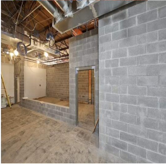
CMU wall completed in kitchen (L)
